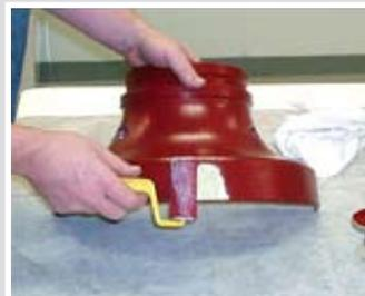
Paint is applied on the primed surface. The paint should slightly overlap the surrounding surfaces.
