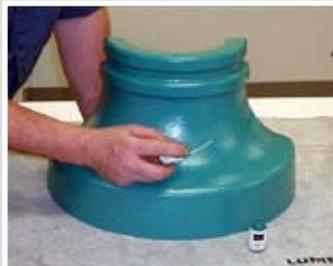
Paint is applied on the prepared surface. The paint should slightly overlap the surrounding surfaces.
